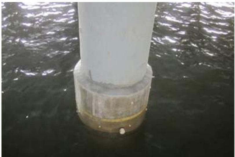
GALVANODE JACKET PORT OF HOUSTON PILE PROTECTION
